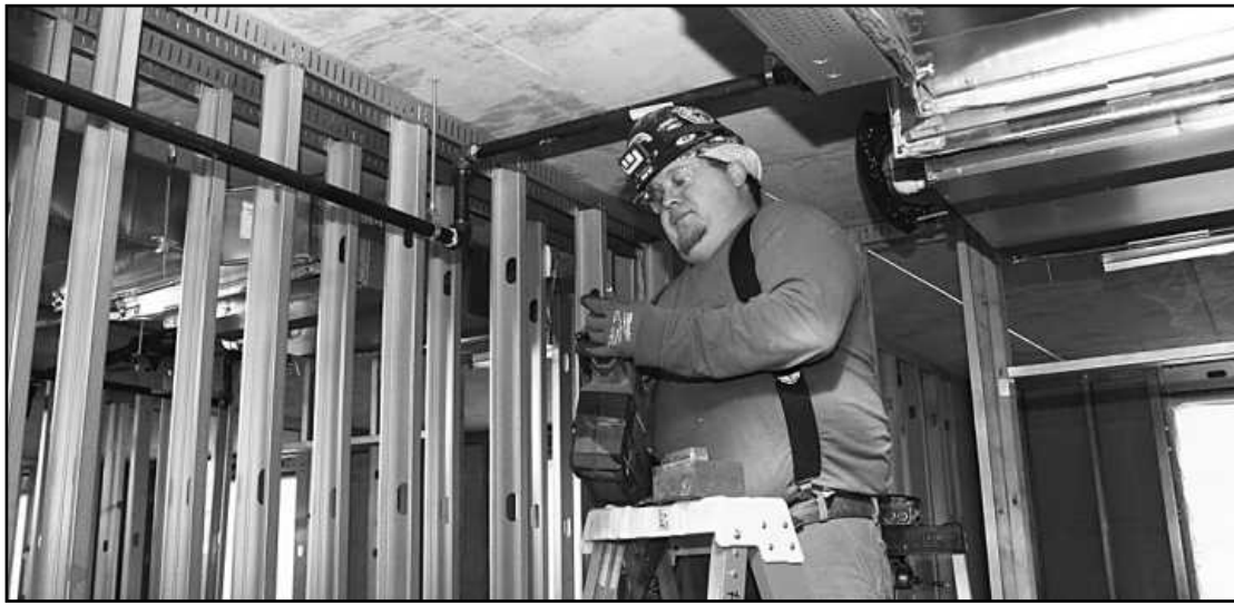
SETTING UP A HAMMER DRILL as he installs fire alarm wiring at the Vanguard Hotel project in Ann Arbor is Dennis Locks of IBEW Local 252. He's employed by Superior Electric.
