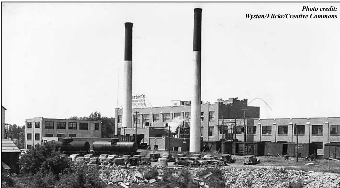
THE GERBER PLANT in Fremont in the 1930s. Today the Nestle-owned campus has grown to be home to the original Gerber factory, the Nestle Research and Development Center for baby meals and drinks, a parent resource center, and several corporate functions such as agriculture, technical applications and procurement.
