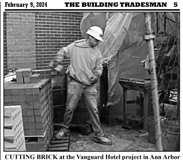
CUTTING BRICK at the Vanguard Hotel project in Ann Arbor is Cody Detlor of Bricklayers and Allied Craftworkers Local 2. He's employed by Leidel and Hart.
