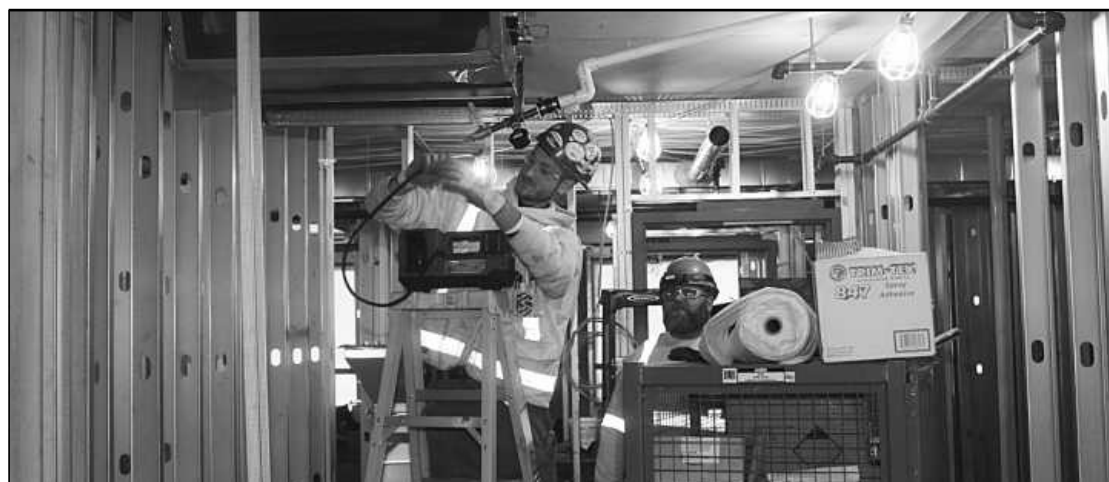
AIR-TESTING PIPE they installed on the fifth floor of the Vanguard Hotel project are Jonah Beisel and Scott Johnson of Plumbers 98. They're employed by Sylvan.
